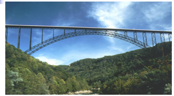
New River Gorge bridge, Fayetteville, WV Main span length: 1700 ft., Built: 1978
