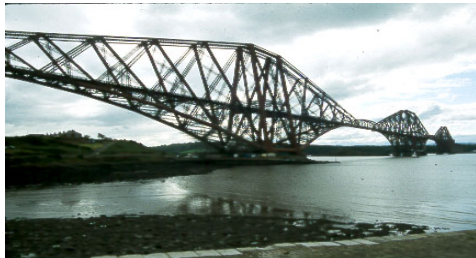
Forth Bridge, Queensferry, Scotland
