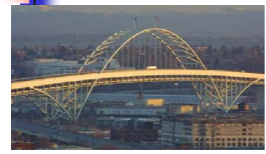
The double-decked Fremont Bridge, Portland, Oregon The tied arch span: 902 feet Built: 1973
